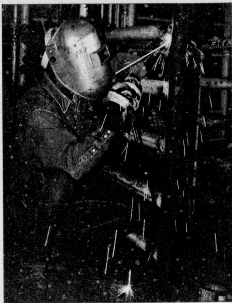
RYON SWINK, A junior agriculture economics major and a member of the Texas Tech Rodeo Association from Crosbyton, welds together a new chute for events such as calf roping, team roping and calf wrestling at the Lubbock Fair Grounds Livestock Pavilion on Tuesday. Swink and others are preparing for the Tech Collegiate Rodeo, which begins Thursday.
