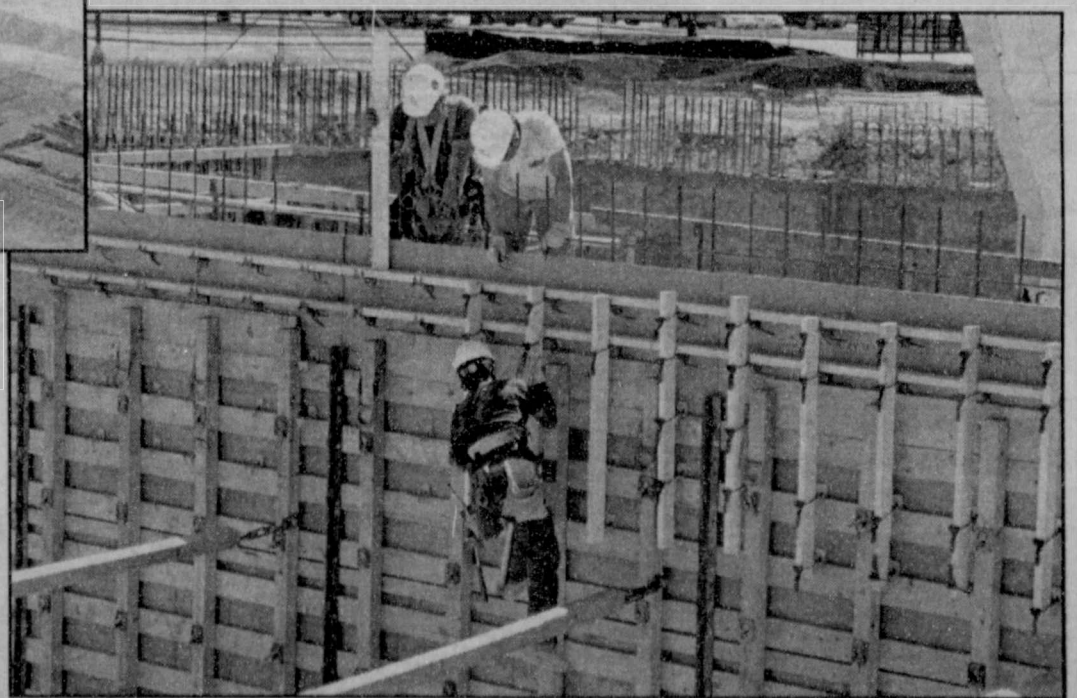
▲ Workers build form work for the basement walls, which will be filled with concrete during the next two weeks.
