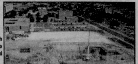
▲ Workers build form work for the basement walls, which will be filled with concrete during the next two weeks.
