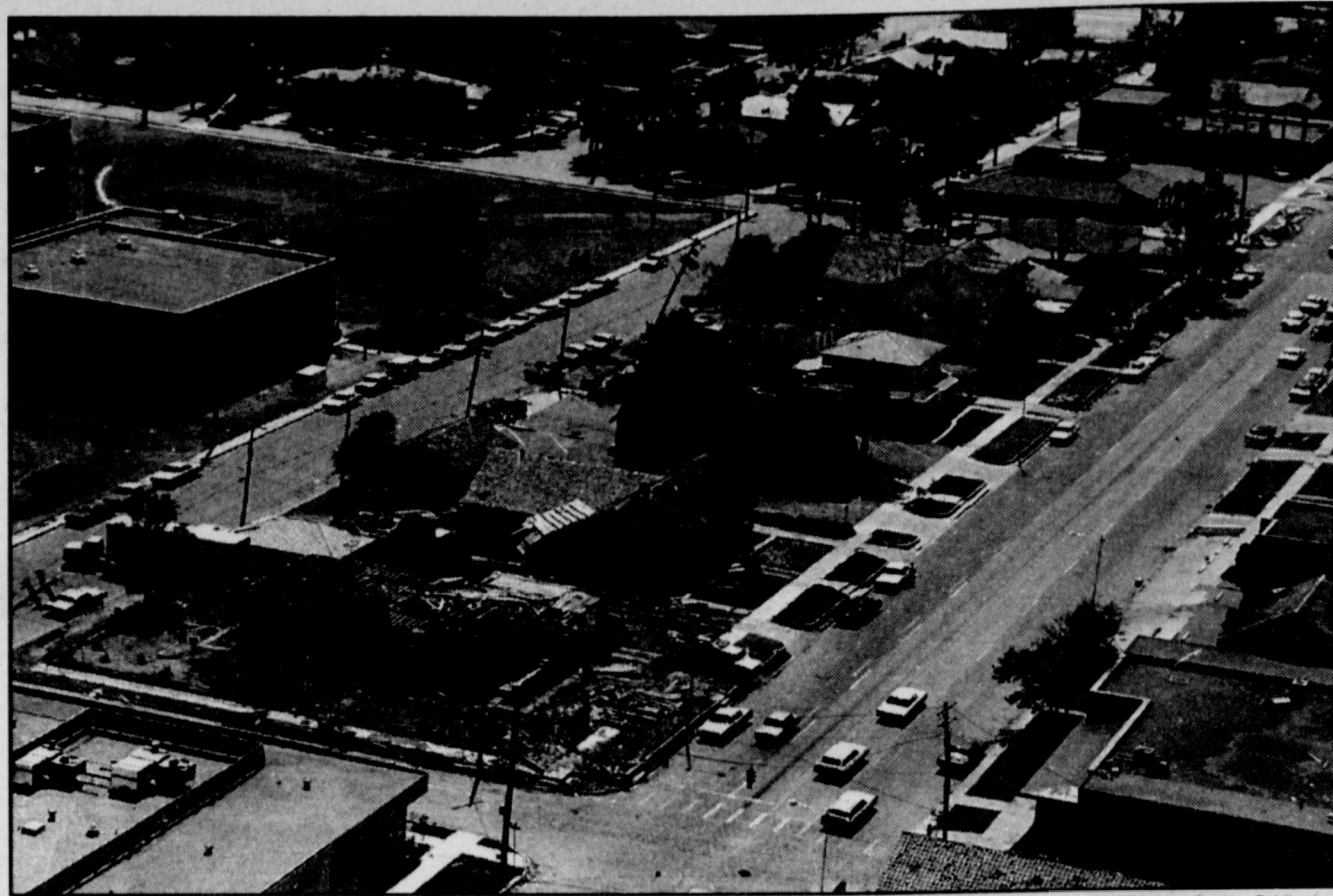
Sporadic destruction can be seen in this photo taken of the aftermath on Broadway from the May 11, 1970, tornado. The devastated house in the middle of the photo is the present location of Gardski's Loft.
