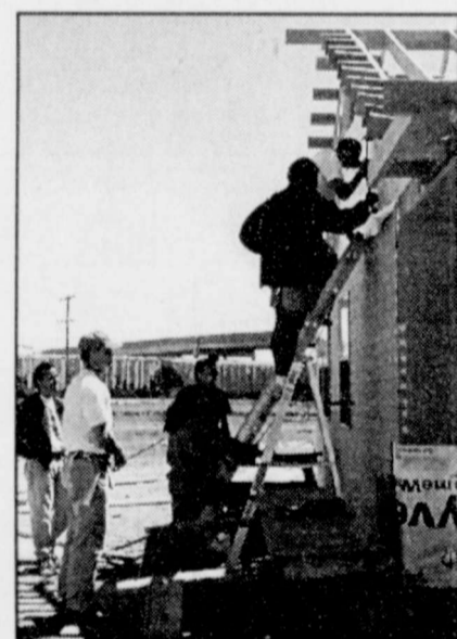
Texas Tech students help build a home.
