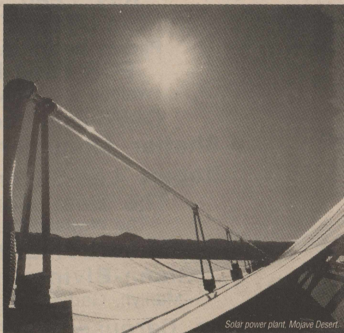
Solar power plant, Mojave Desert.
