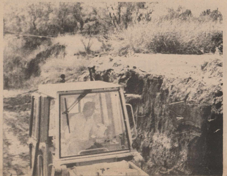
Jesse Torres, Coke County employee, at work finishing deep cut across Exxon Road on Rough Creek to accommodate a 56' long railroad tank car converted to a tinhorn to take care of runoff water in the steep draw.
