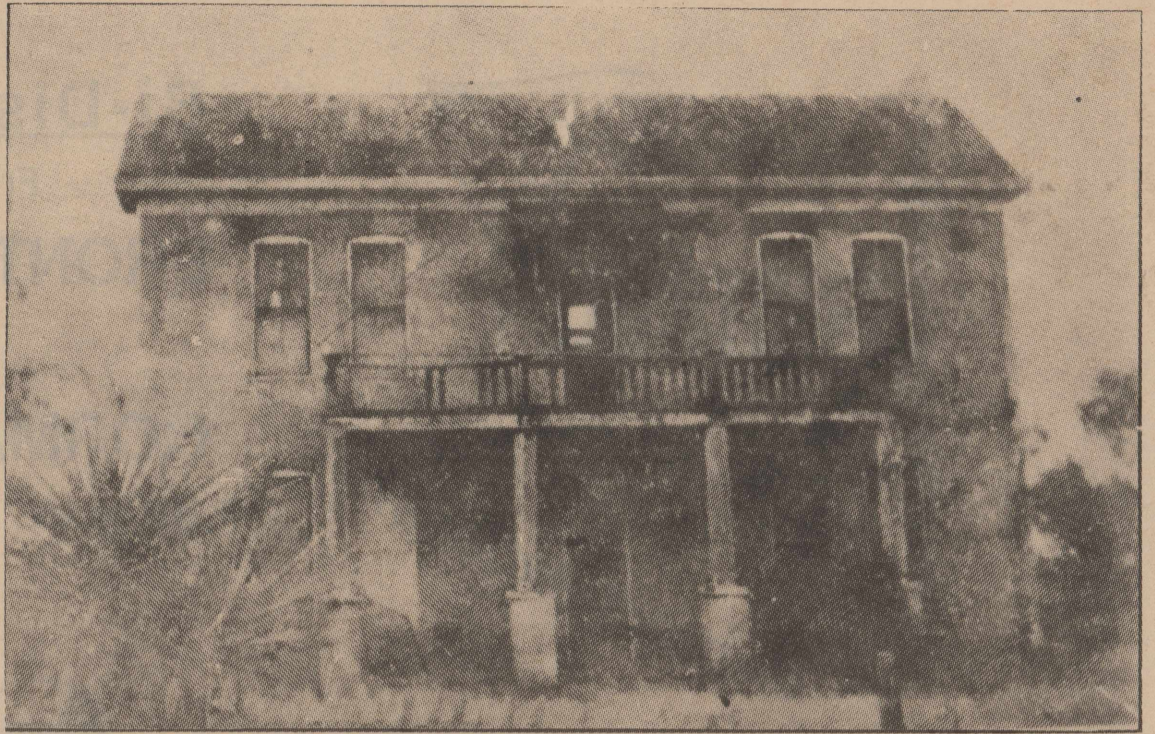
The historic Harris Ranch headquarters was located just south of the Colorado River near Robert Lee. It was constructed of adobe bricks made in a pasture on the ranch. A landmark in Coke County, it stood nearly a century before being gutted by fire in 1945. (Picture courtesy of Jewell Pritchett.)
