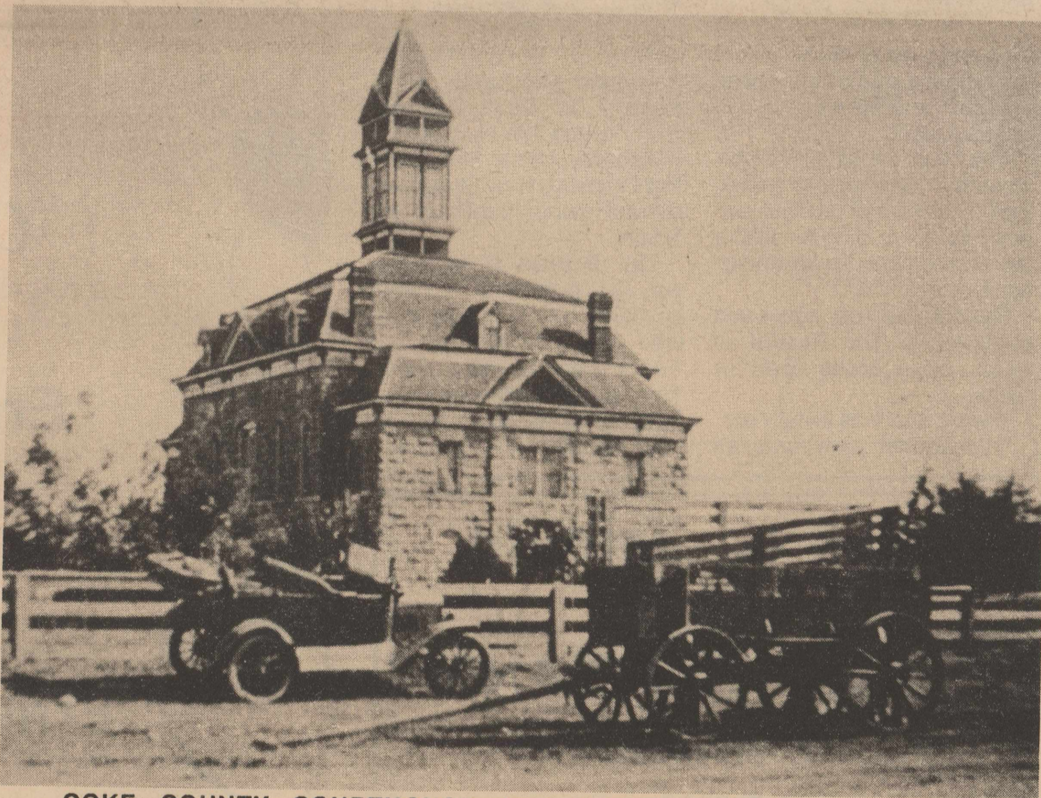
COKE COUNTY COURTHOUSE 1891-1956. In the Spring of 1891 the cornerstone was laid for the Courthouse that was to be the home of Coke County Records and Law Officials for Sixty-five years. Built of native stone quarried by hand, most of the stone came from the Kirkland Ranch, and was hauled in wagons.
