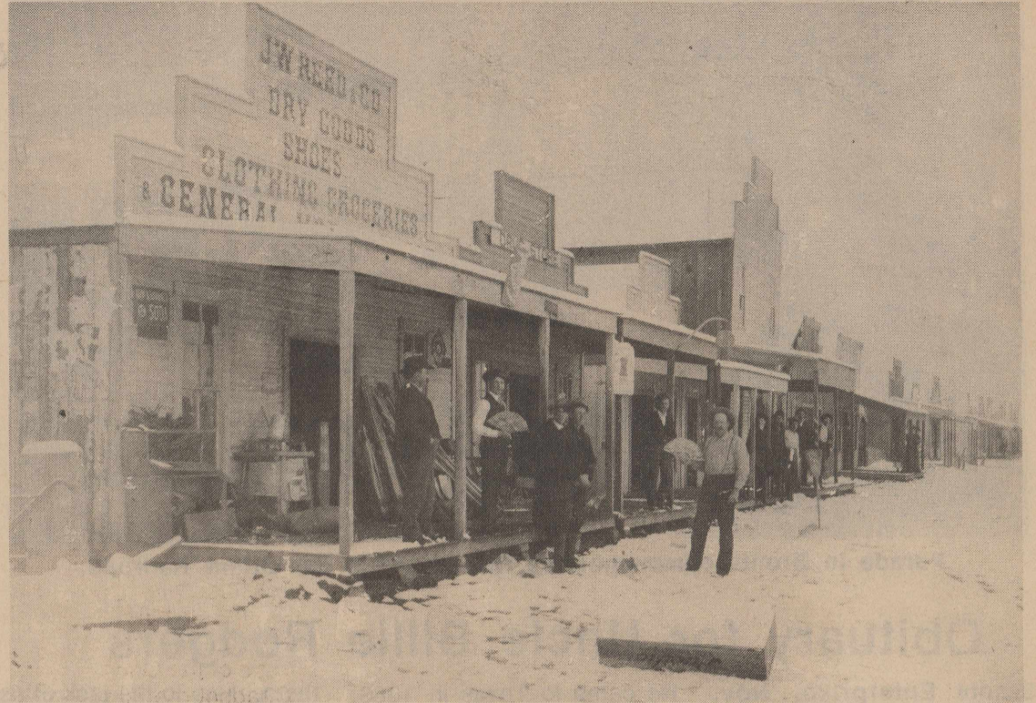
J. N. K. Adams, part-owner of J. W. Reed and Company, stands in the street fanning himself, with snow on the ground, 1901. Business was located on west side of Austin Avenue. South side of the building was blown out a short time later when Jim Clift accidentally dropped his cigarette in a barrel of gunpowder. Luckily no one was injured. Tall building near middle of the block was the Woodmen of the World Lodge.
