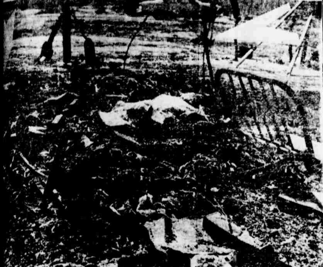
Remains were all that was left of the farm home destroyed Sunday morning in a sudden fire. The family lost everything it owned—cash, clothes, furniture—before anyone could arrive to help. Arrow at right indicates the stove that exploded; arrow at left the parents' bed. (Abilene Reporter-News photo by Wm. E. Stanfill)
