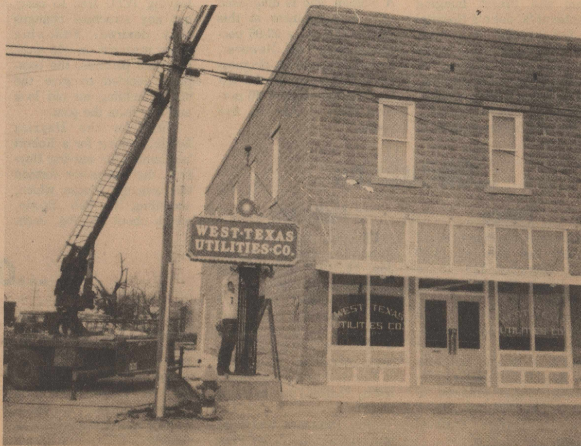
BOB BOONE, LOCAL WTU manager, assists a West Texas Utility construction crew in setting the handsome "new" sign outside the Robert Lee office. It is part of the renovation and sprucing up of the historical site. [related story inside]
