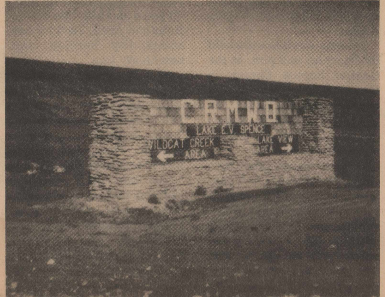
ATTRACTIVE NEW SIGNS are being placed at entrances around Lake Spence as the lake personnel's recreation crew is available for the construction. They are doing a beautiful job with native rock from the Divide donated by Ethel Harmon and Dennis Counts from their ranches, and combined with cedar-type shingles.
