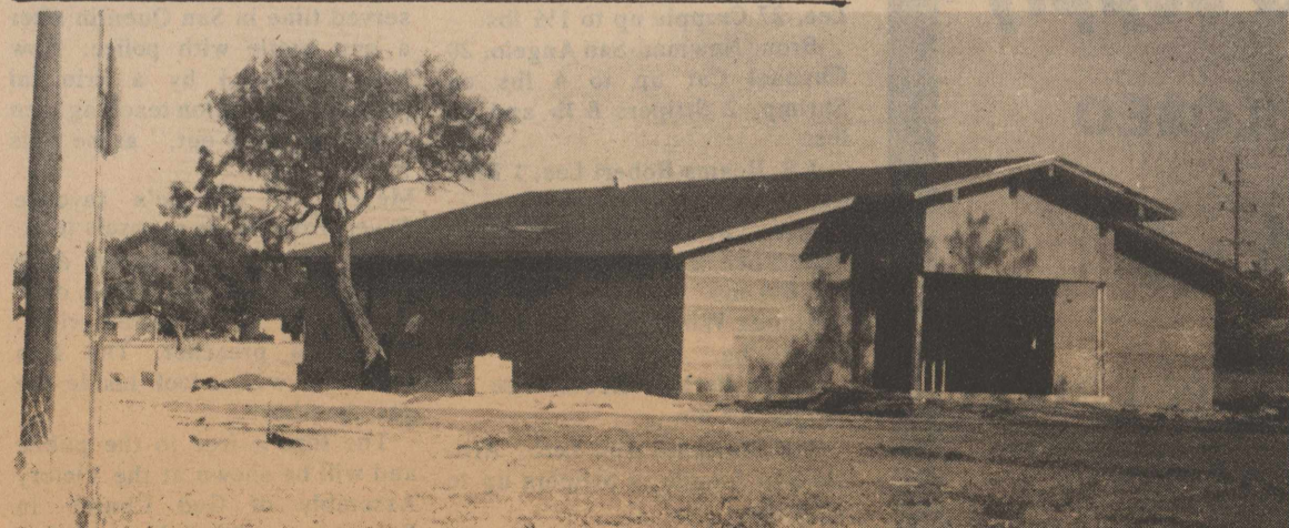
Work Continues On New Post Office Building
