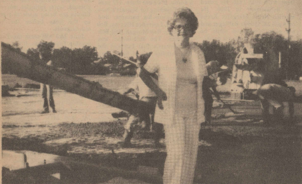
ROBERT LEE POSTMISTRESS Coe Lewis surveys the site of the new Post Office building at 6th and Houston in Robert Lee.
