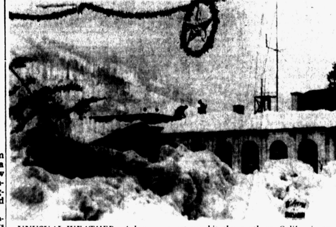
UNUSUAL WEATHER—A heavy snowstorm hit the northern California town of Dunsuir this week and before it ended the town and its 3,700 residents were without electricity for two days. Then it started to rain and buildings collapsed. Here men are busy shoveling snow from the top of a downtown building. Decorations still hang to remind the citizens there had been a Christmas. (AP Wire-photo)
