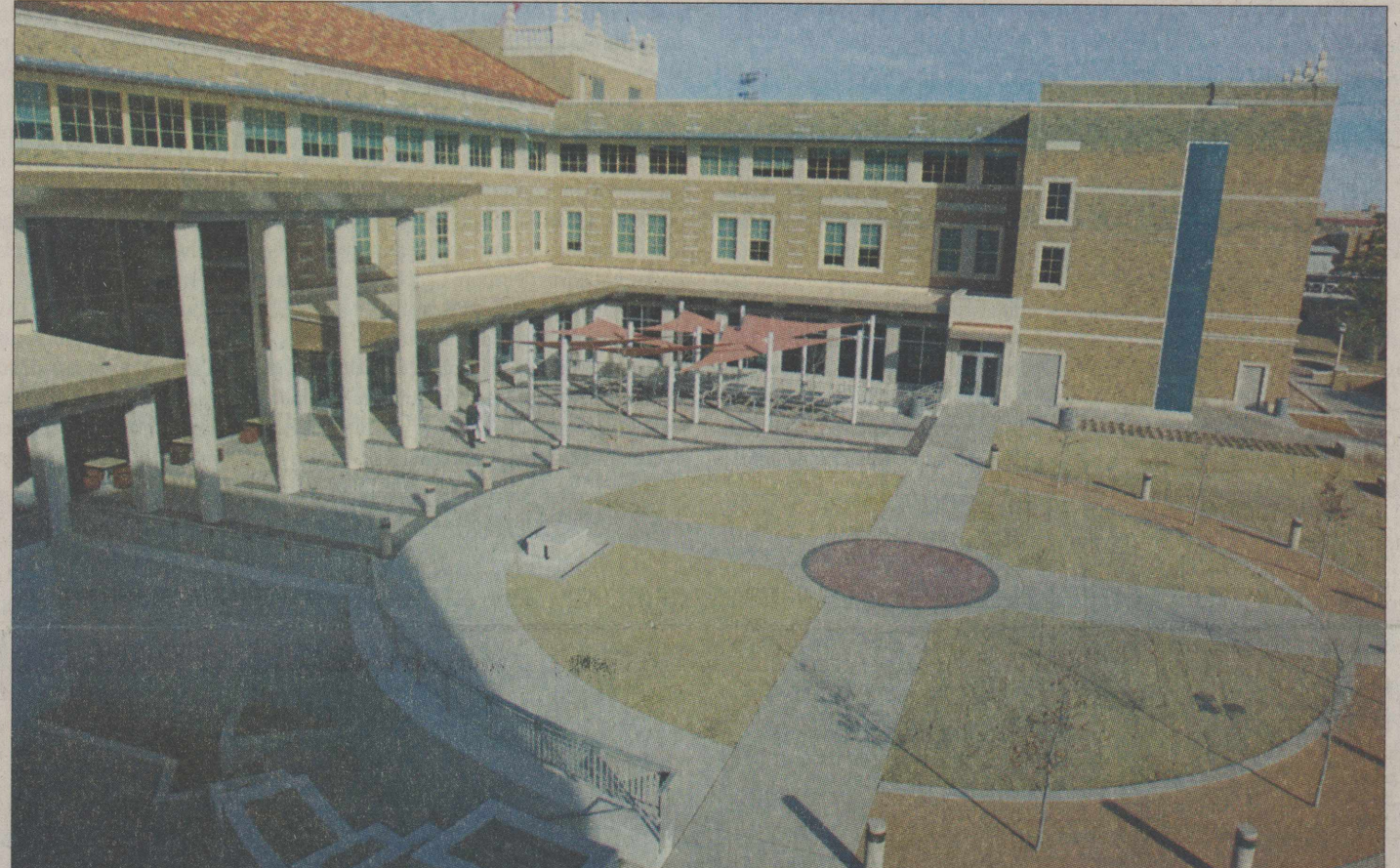
CONSTRUCTION ON THE new Rawls College of Business Administration building is complete and is open for classes starting this semester.
