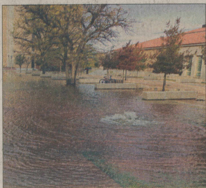
PHOTO BY BRAD TOLLEFSON/The Daily Toreador WATER FLOWS OUT of a broken water main between the Experimental Science building and Science building Saturday morning.
