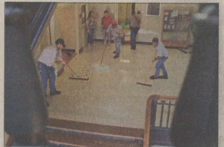
PHOTOS BY BRAD TOLLEFSON/The Daily Toreador PHYSICAL PLANT EMPLOYEES sweep water down the main stairway in the Math building after a pipe burst flooded the first floor of the building Friday. Approximately 20 workers were on site to take care of the water.
