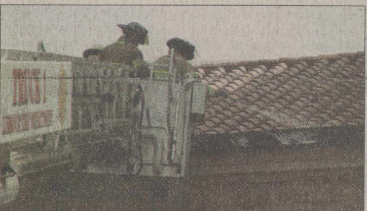
THE LUBBOCK FIRE Department was called when a fire was reported in a gutter on the roof of Stangel/Murdough Residence Complex on Monday. No injuries or damages were reported.
