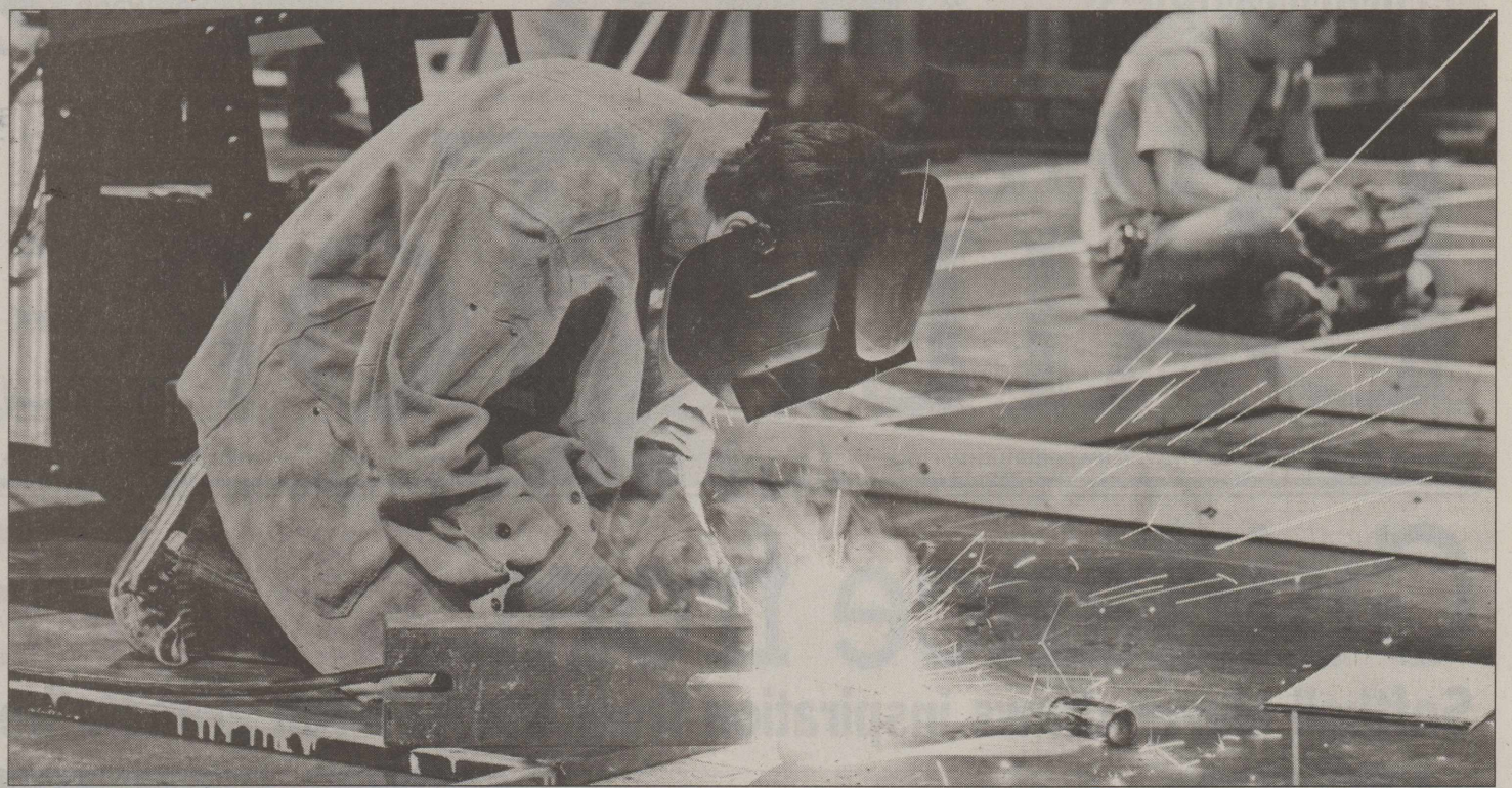
PHOTO BY SAM GREINADIER/The Daily Toreador SARA STRIBLING, A senior theater design major from San Antonio, welds a metal frame together for the set of the upcoming musical “Curtains” Tuesday in the Charles E. Maedgen Jr. Theatre.
