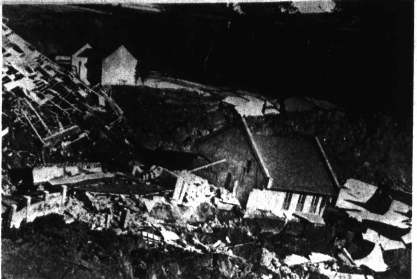
Buildings and greenhouses were destroyed on Jefferson Island, La., last Thursday after a drilling rig punctured a salt mine shaft 1300 feet below the surface of Lake Peigneur. Inspectors are trying to piece together exactly what happened in the incident of the cave-in that has left 250 salt miners out of work.
