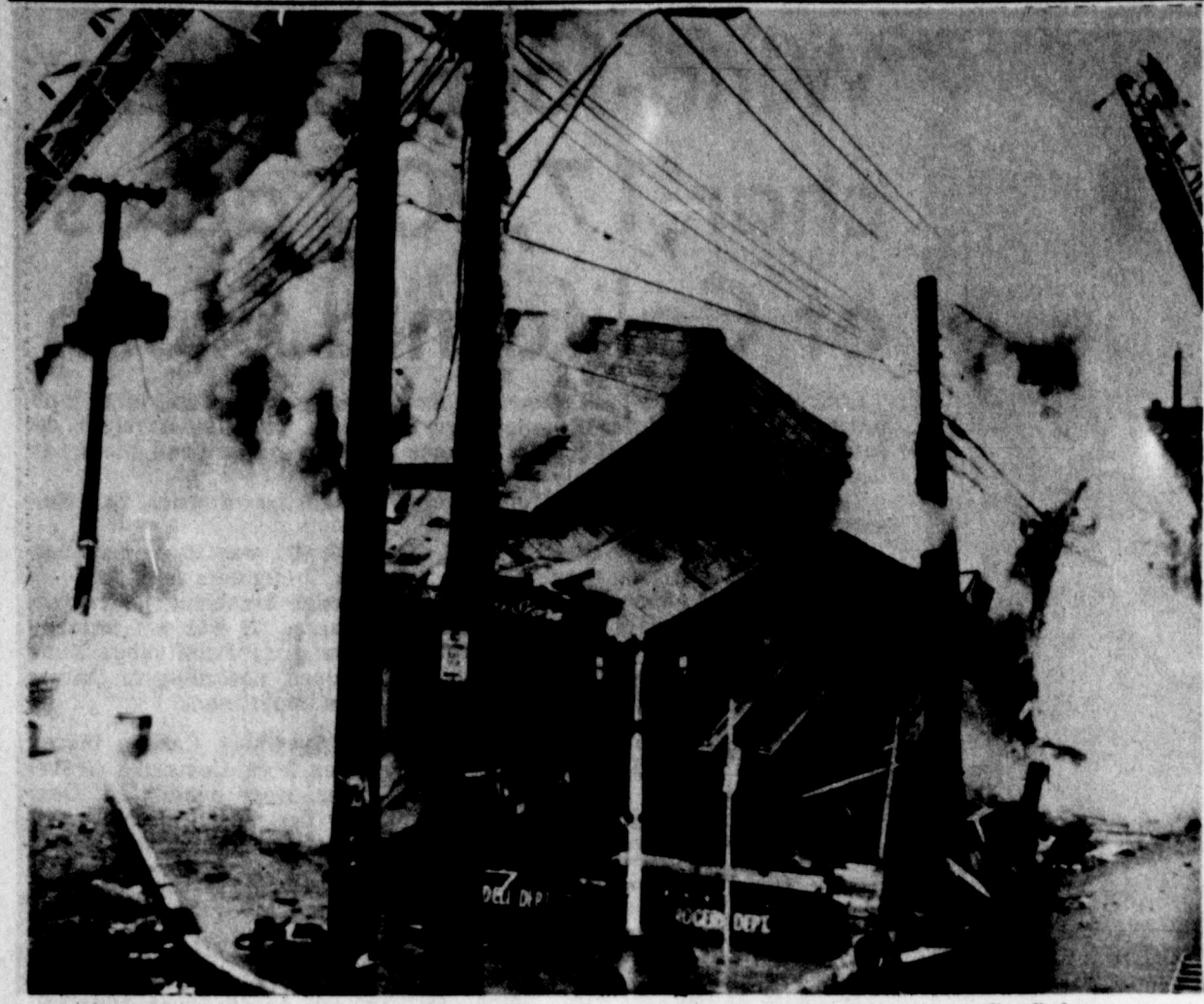
A two-story structure at Yonkers Avenue and Bronx Road, in Yonkers, N.Y., collapses Tuesday after a three-alarm blaze
