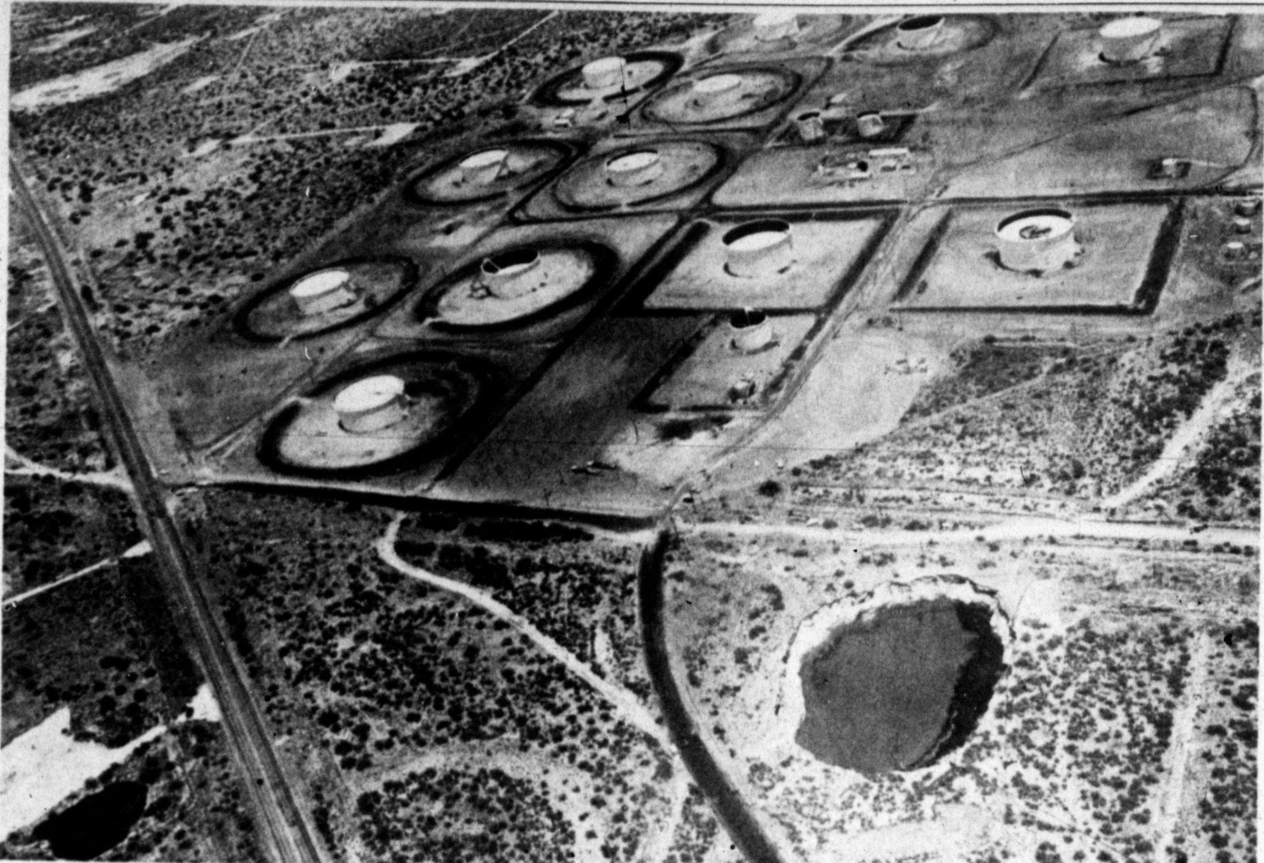
Measurements show the Kermit "crater," bottom right, to be slowing in its growth toward a Shell Oil Co. tank farm and State Hwy. 115, shown running diagonally at the far left. As of this morning, according to officials at the site, the hole was within 300 feet of the highway and 1,110 feet of the tank farm. (Staff Photo by Bruce Partain)
