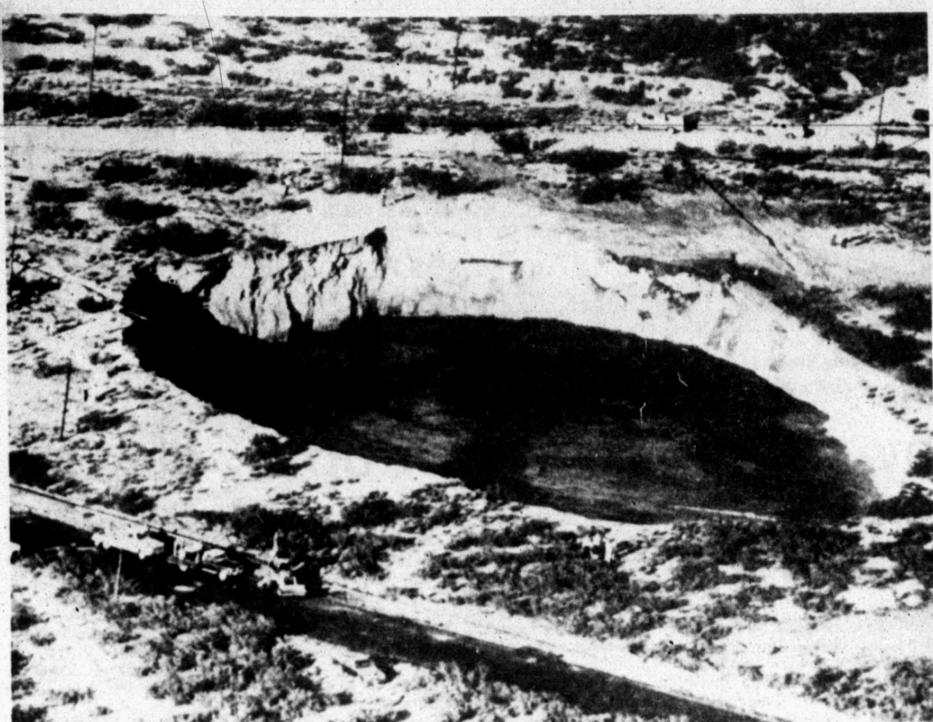
An aerial view from 400 feet shows the growing sinkhole near FM 115 between Kermit and Wink. When this photo was taken Wednesday, the crater was measured at 50 by 100 yards, but by early today it had grown to approximately 200 by 250 yards. See related photo, Page 2A. (AP Laserphoto)
