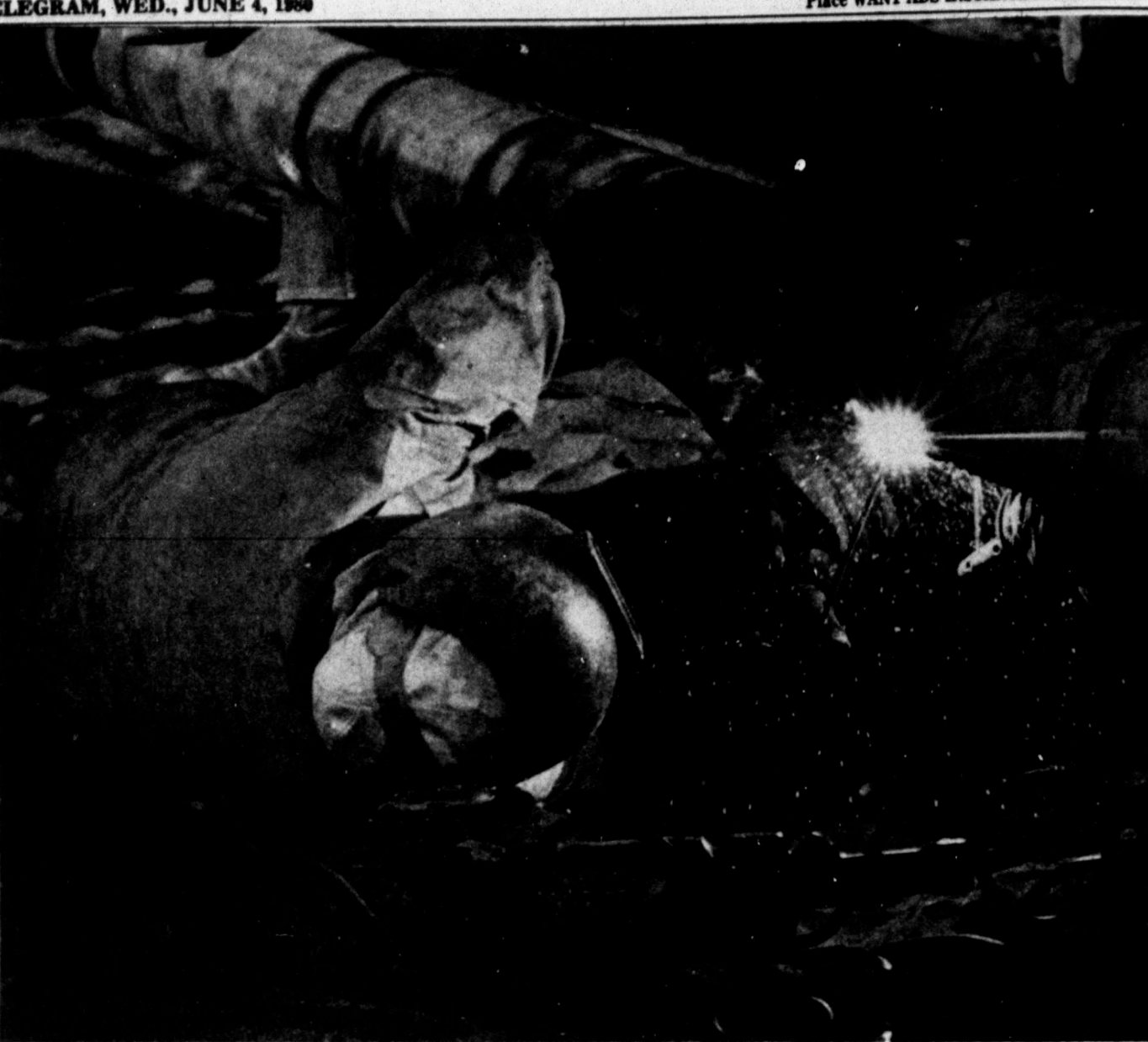
A Shell Oil Co. welder works on a pipeline near the growing sinkhole southwest of Kermit. At least one crude oil and one water line were broken when the ground collapsed near a Shell tank farm Tuesday, and employees worked to move other lines away from the pit. (Staff Photo by Bruce Partain.)
