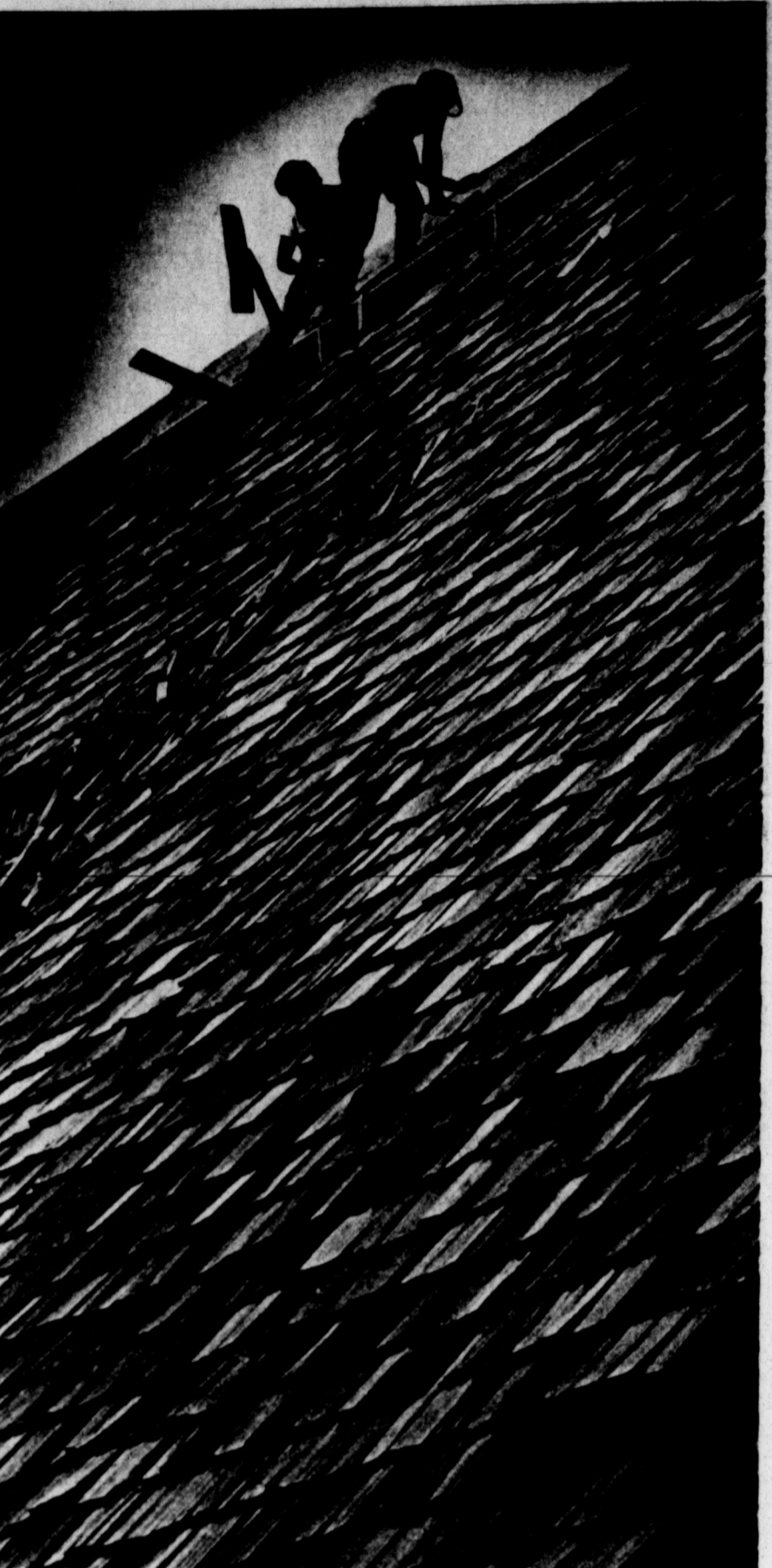
Getting into a steep situation, David Gonzales and Robert Aldana, employees of a local roofing company, tear old shingles from the roof of Bellview Baptist Church on North Big Spring Street. The roofers expect the reroofing will take several days and several thousand shingles to complete. (Staff Photo by Brian Hendershot)
