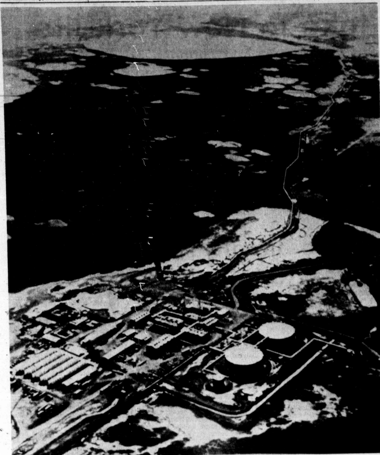
Photo shows Pump Station One at Prudhoe Bay, Alaska, where crude oil begins its 800-mile journey through the trans-Alaska pipeline to the southern terminus at Valdez, in June, 1977. Three years after oil began flowing through the controversial pipeline, Alaska is beset with economic benefits and environmental and governmental problems. (AP Laserphoto)
