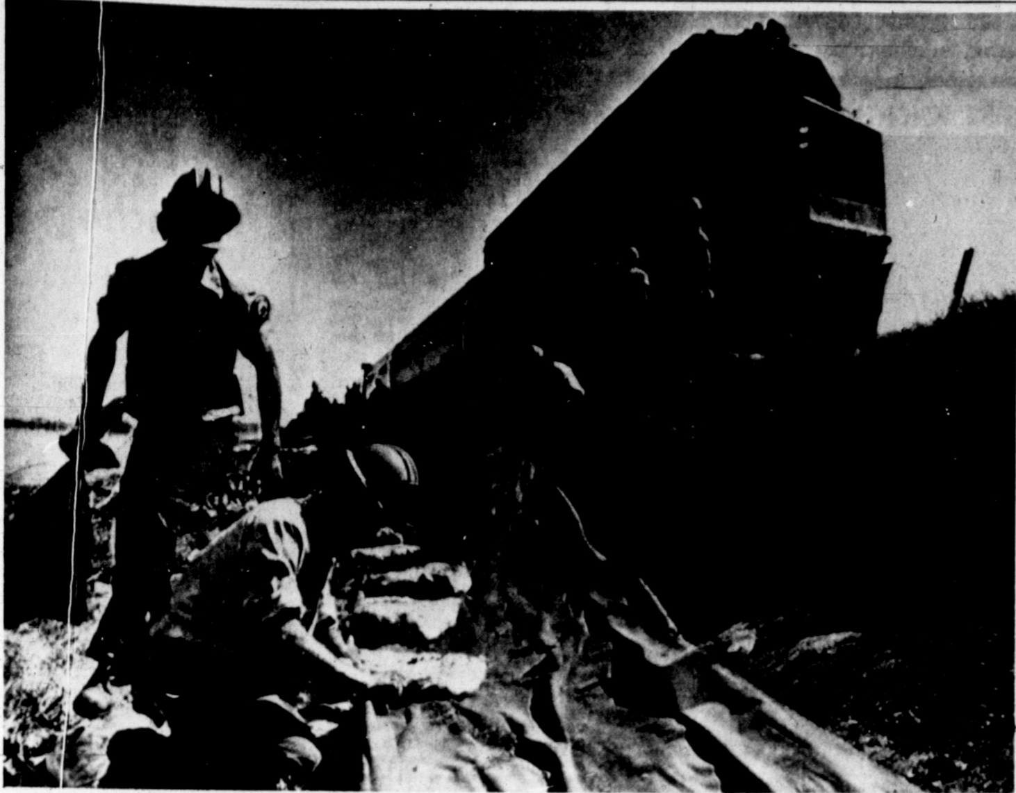
Some of the more than 200 California Conservation Corps workers place sandbags and sheathing along a weakened Santa Fe Reailway levee 10 miles west of Stockton
