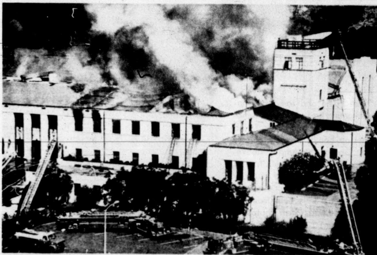
Firefighters battle for control of a fire which badly damaged the two-story Naval and Marine Corps Reserve Center in the Elysian Park area of Los Angeles Saturday. One fireman died and four others were injured, according to a city fire department spokesman. (AP Laserphoto)
