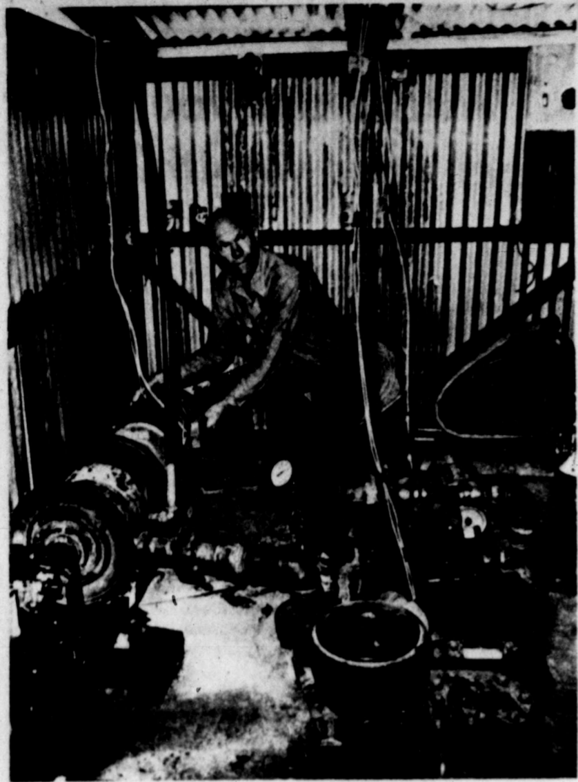
Homer Peterson, 70, works in a shed behind his house in Middletown, Calif., with a hydroelectric system his dad installed in 1907 when he got tired of candlelight. On the left, hidden in a housing flanked by two Model T Ford flywheels is a water wheel that is spun by water running through a pipe from two reservoirs on the Peterson ranch, thus turning the generator. (Los Angeles Times Photo by Charles Hillinger)
