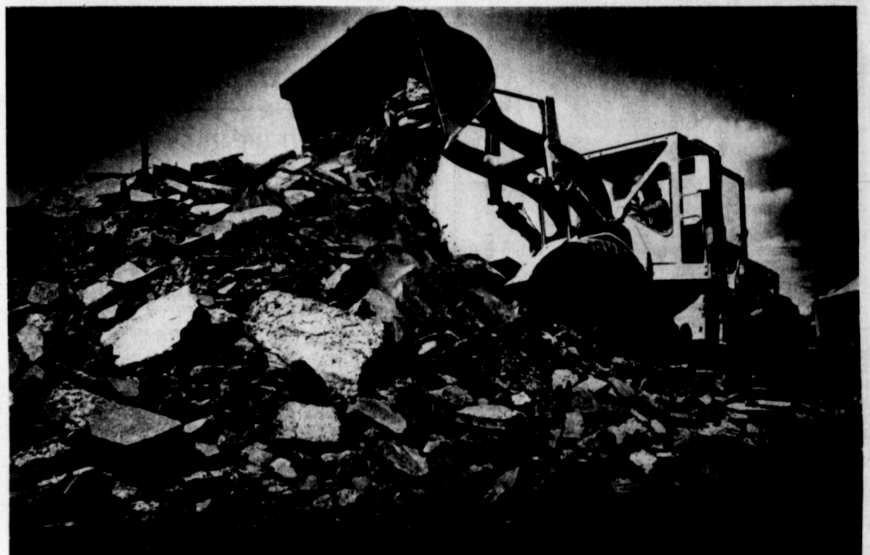
What used to be a several-block stretch of Midkiff Road lies in one large pile with the machinery throwing on more of the crushed street. The city started work Monday on a $1.3 million project to rebuild Midkiff Road from Illinois to Storey streets. The final project will go north to Golf Course Road and include the intersection at Illinois. (Staff Photo by Brian Hendershot)
