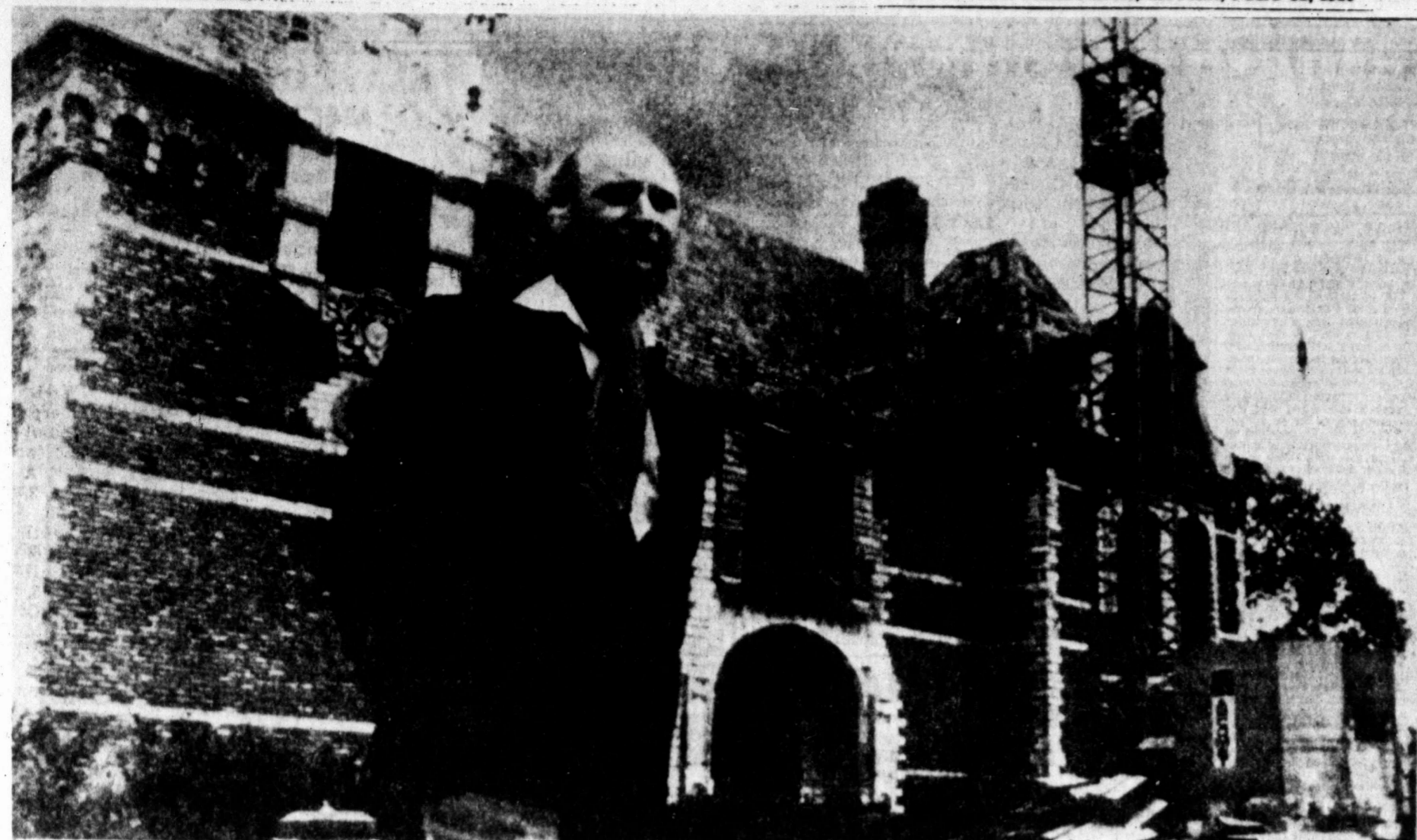
Architect Marcel Raymaekers stands in front of a home he recently designed in Hasselt, Belgium, from materials recycled from castles. Raymaekers says, "For me, the historical value of the places we tear down is the least important." (AP Laserphoto)
