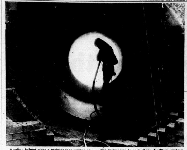
A safety helmet gives a maintenance worker at PPG Industries' Lake Charles, La., chemicals complex an astronaut's appearance as he cleans a waste incinerator with sandblasting equipment.
