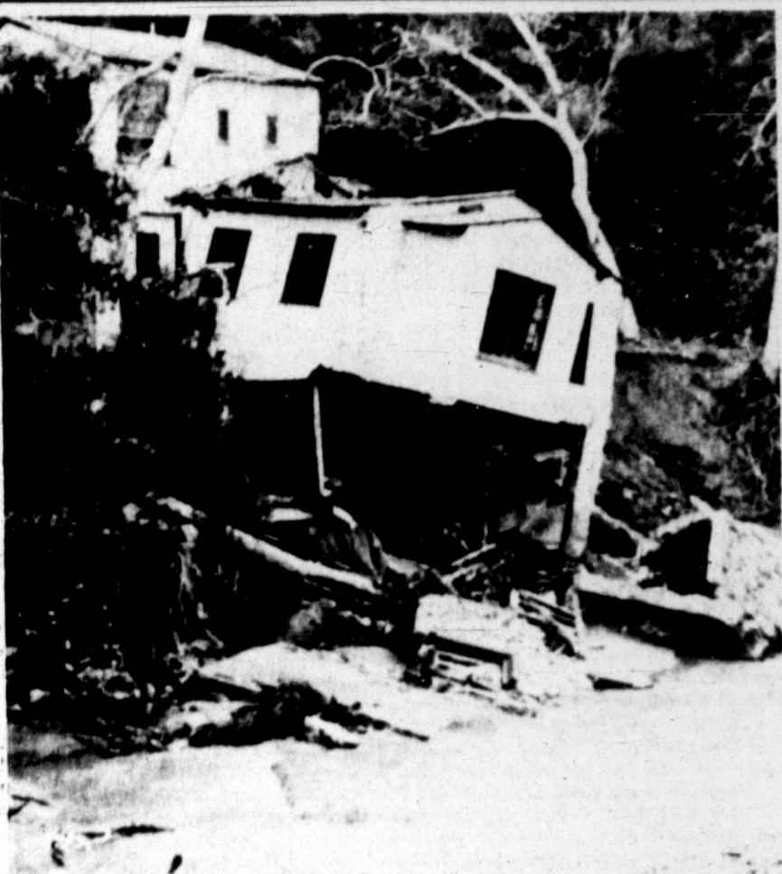
A house stands ready to topple beside floodwaters in Topanga Canyon section of Los Angeles Wednesday. A series of Pacific rainstorms caused severe flooding and mudsliding throughout much of southern California. Many homes have been destroyed by the rains. (AP Laserphoto)
