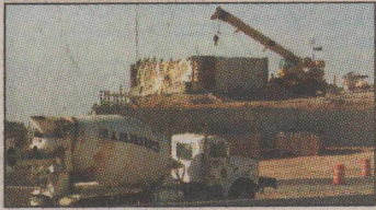
CONSTRUCTION UPDATE SEE PAGE 8
