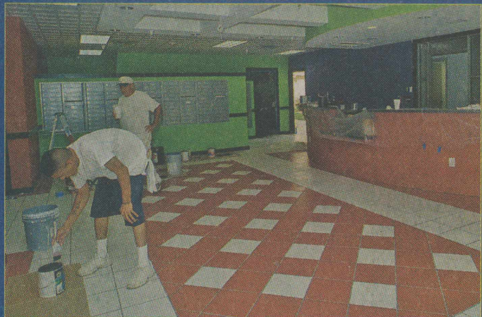
EMPLOYEES PAINT SECTIONS of U Lofts to prepare for Thursday's inspection.
