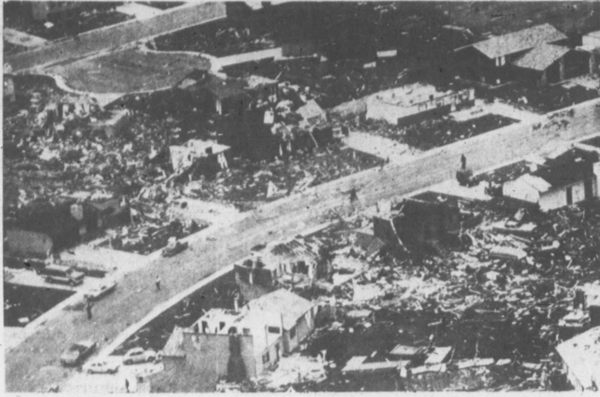
This aerial photo shows tornado damage to the Buffalo Ridge area of Cheyenne, Wyo.
