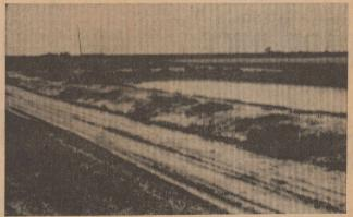
Tail water recovery systems like this system on the J. D. Nance place help farmers get the most use out of their dwindling supply of irrigation water. Many farmers have found that they get more water out of a recovery system than they can get from a new well.
