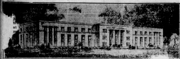
Construction work has started on a new three-story building to house the Agricultural Adjust-
