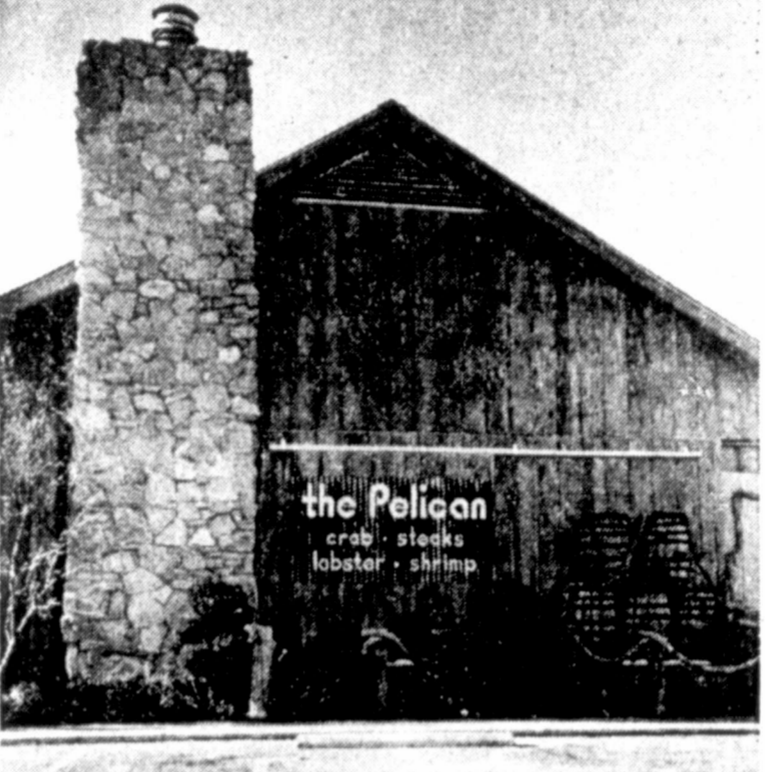
LATCHSTRING OUT AT LOOP 289 AND INDIANA
