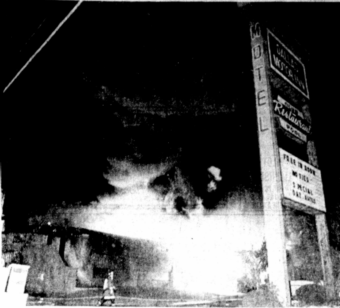
HOTEL BLAZE — A five-alarm fire caused heavy damage Wednesday night when it swept through the two-story Dallas Motor Inn. Two persons were reported injured in the fire that engulfed the whole building. The fire department said 18 pieces of equipment and about 80 men battled the blaze. (AP Laserphoto)
