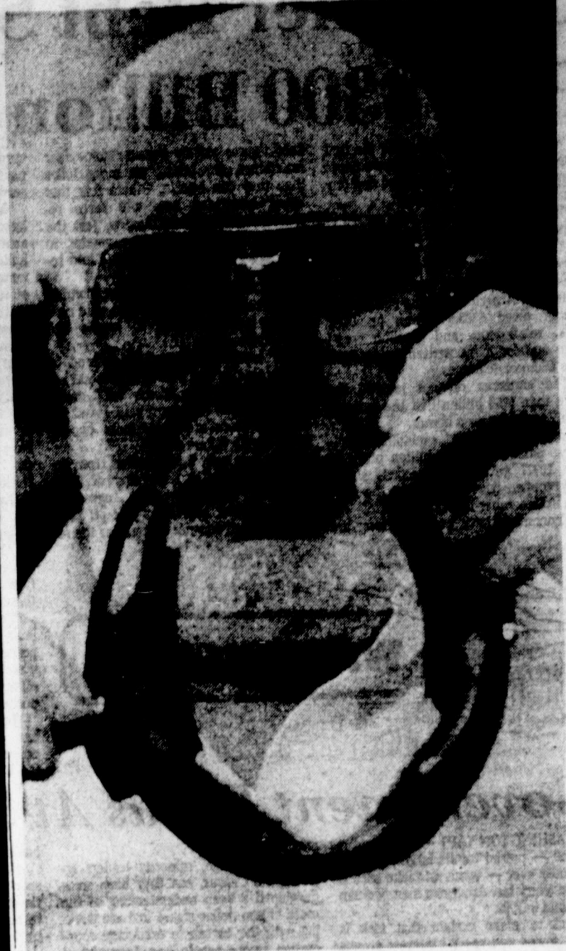
SNORE CURE — Robert Crossley of Austin, a reformed snorer, shows his patented snore cure. The vinyl-covered collar is equipped with a microphone that picks up the sound of snoring. The collar then throws a mild shock into the snorer's neck. Works almost every time, Crossley says. (AP Laserphoto)
