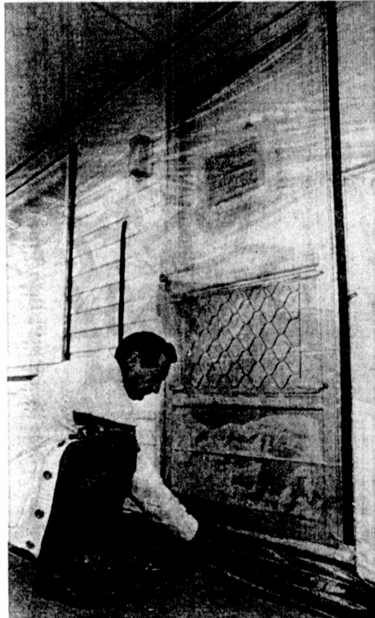
PLASTIC WRAP — Richard Ammerman of Perrysburg, Ohio, adjusts the plastic he has used to wrap his house for the winter. The northwestern Ohio homeowner left only his backdoor uncovered in an effort to stop winter drafts. (AP Laserphoto)
