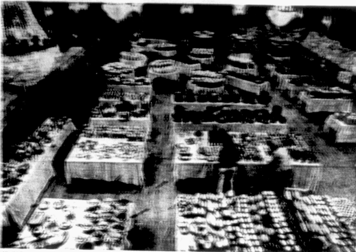
UPPER BALLROOM — This is the ballroom of the Baker Hotel in Dallas, once the scene of fancy parties and dances, now a huge ballroom for the hotel's remodeling. The building is to be demolished and all contents from knives and forks to the crystal chandeliers are up for sale. The sale open to the public, starts Wednesday and will run for 45 days. AP/Laserna
