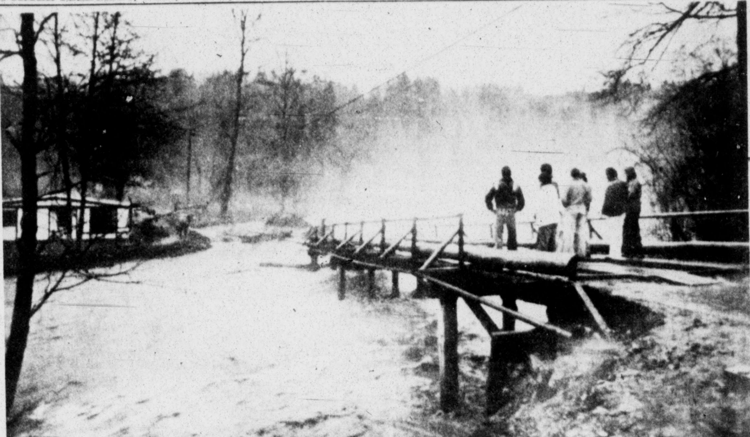
Clallam County, Wash., residents look at the remains of a bridge that was partly washed away when Morris Creek overflowed Monday. Gov. Dixy Lee Ray has declared a
