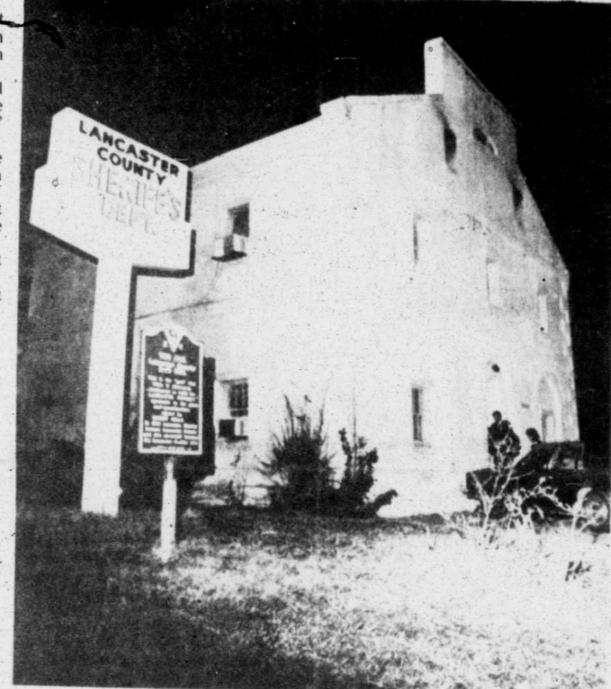
Three men died in the cell pictured above when fire swept through the top floor of the 156-year-old Lancaster County Jail building on the left. In all, ten inmates trapped behind bars died during the fire and autopsy results all died of smoke inhalation. A padlock that failed to open and a wall of heat and smoke prevented rescue of the inmates, officials indicated. (AP Laserphotos)
