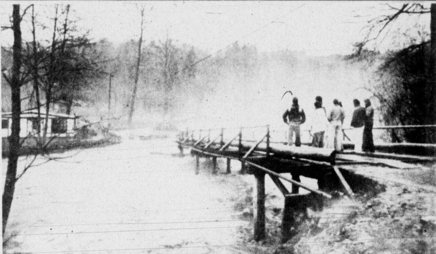
Clallam County, Wash., residents look at the remains of a bridge that was partly washed away when Morris Creek overflowed Monday. Gov. Dixy Lee Ray has declared a state of emergency as winter rains caused flooding in western Washington and the Olympic Peninsula areas. (AP Laserphoto)
