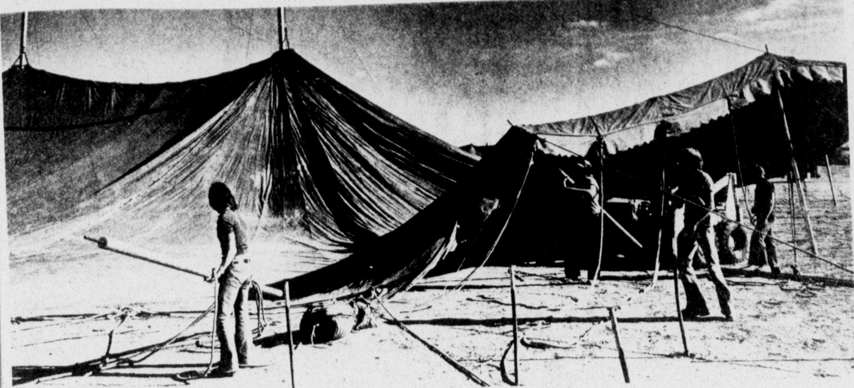
Once the outer edge of the tent is staked with 12-foot poles, crews will winch the canvas about halfway up the main masts before job. bringing in the elephants to help finish the
