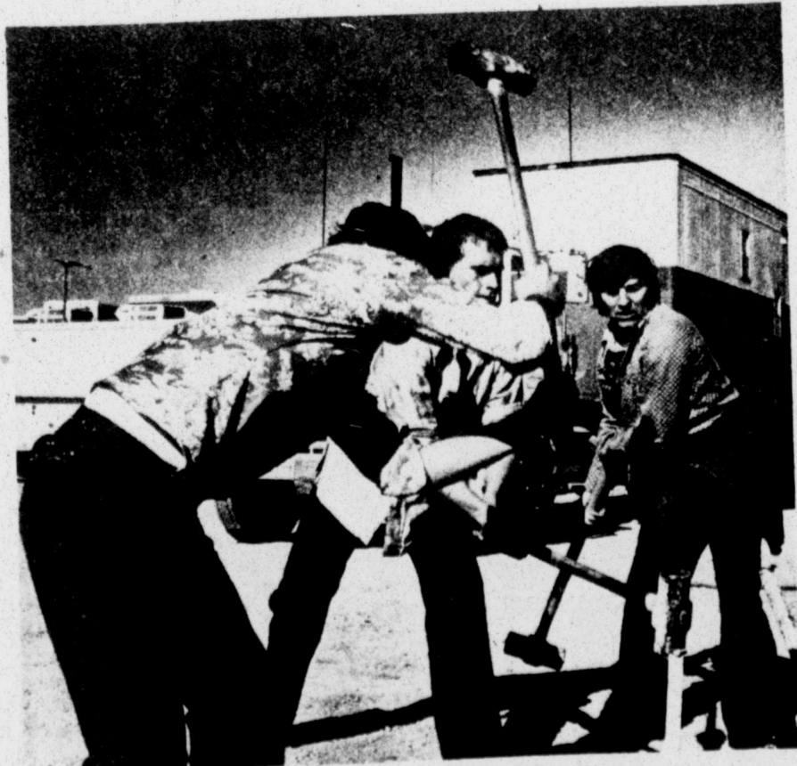
Some of the metal stakes must be driven into the ground the hard way, but coordinated effort works faster, and also creates a unique rhythm.
