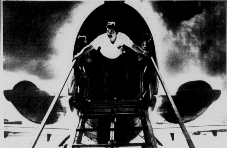
An Eastern Airlines mechanic exits the aft section of a DC-9 after preparing it for a federally-ordered inspection in Miami, Fla., Wednesday. Airline inspectors are checking for cracks in the aft bulkhead, an emergency exit door jamb and bulkhead skin. (AP Laserphoto)
