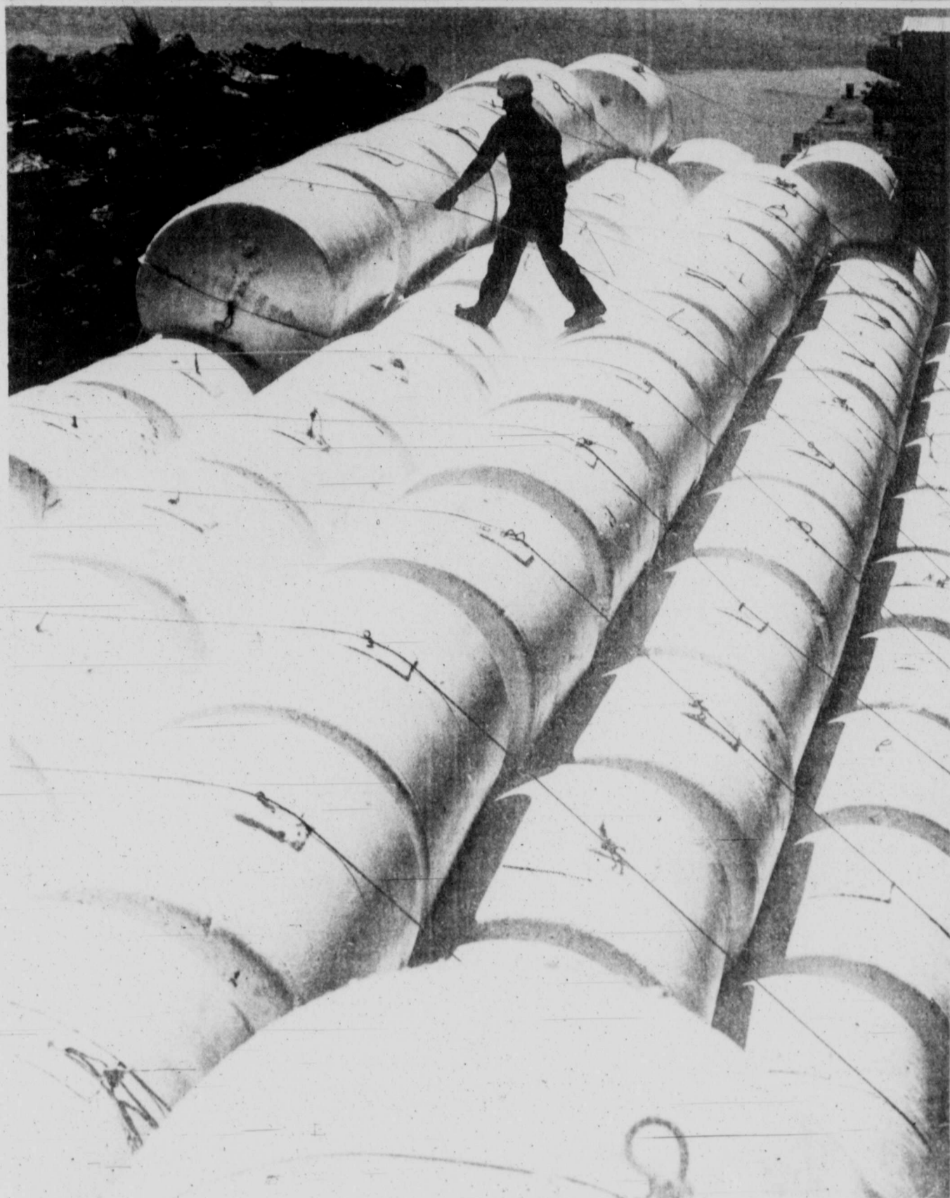
Floatation vocation. That is what you could call Nolan Breaux's job in the marshlands of south Louisiana. These plastic foam devices, looking like large picnic coolers, are used by Tenneco's Tennessee Gas Pipeline Co. in marshland construction. A
