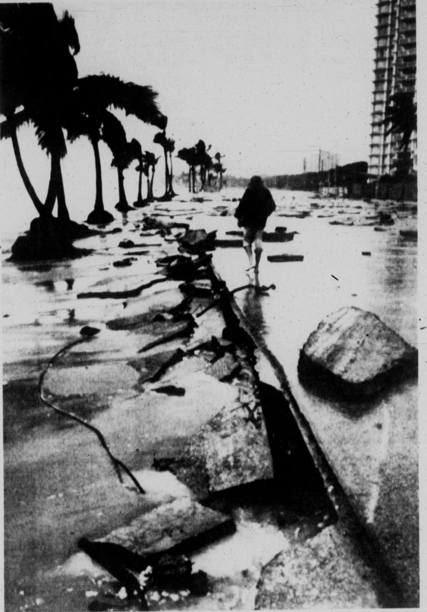
Pavement torn apart by the pounding surf produced as Hurricane David hit the area is seen along the Fort Lauderdale beach. The storm is moving northward up the Florida coast, much weaker than it was when it caused extensive damage in the Caribbean. (AP Laserphoto)
